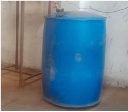
Fig 3 Digester tank during Digestion
