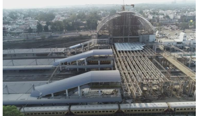
Fig. 3 Steel work in station
