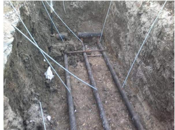
Figure-2. Placed buried tube inside earth
